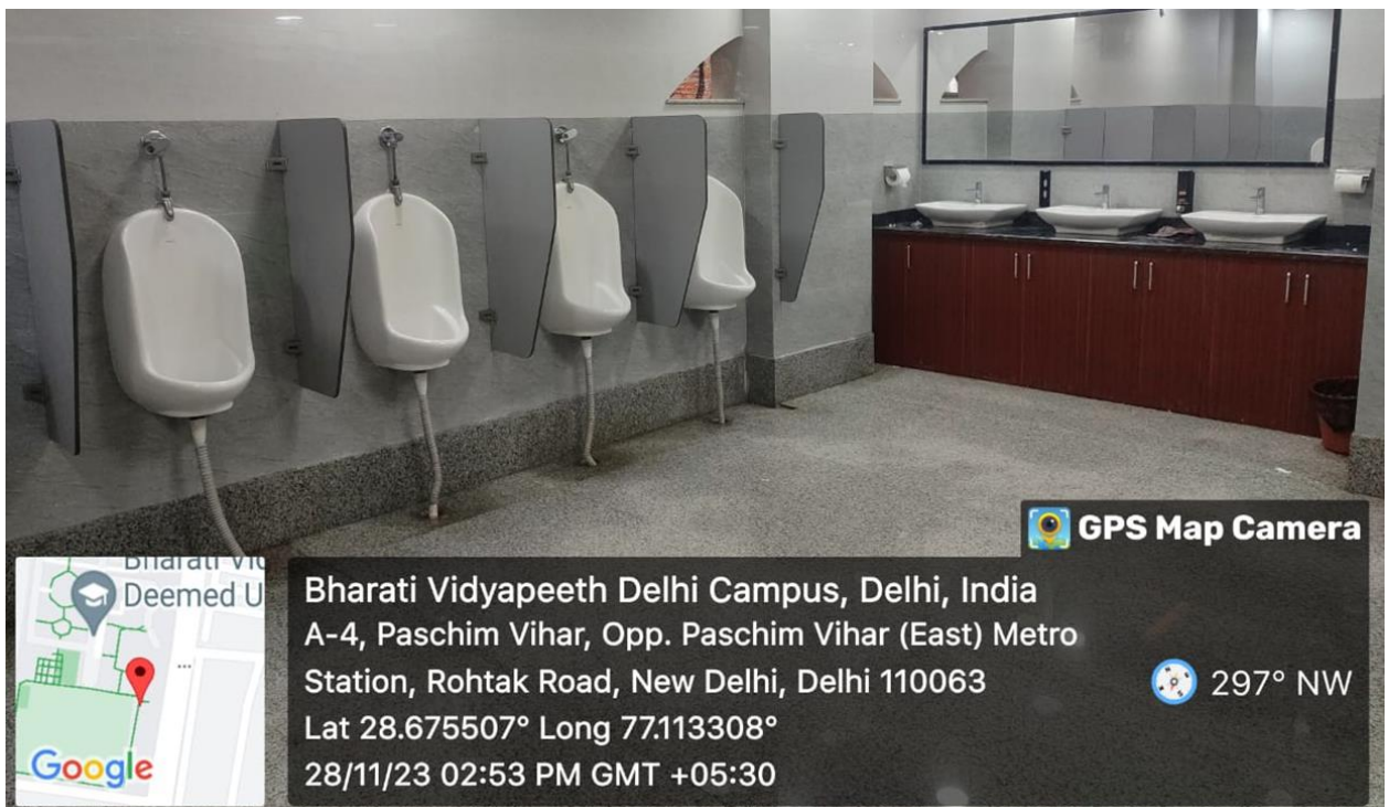
Photo: Cleanliness of toilet
